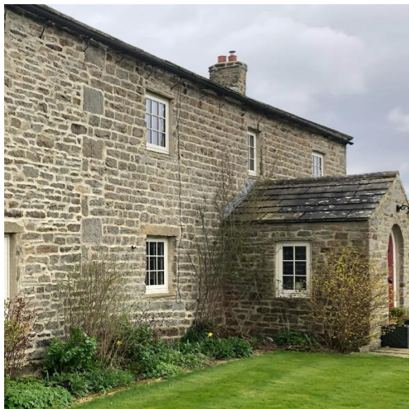
Figure 2 - Typical older, stone built property
