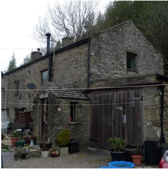
Figure 18 - Older, stone cottage in Richmondshire
